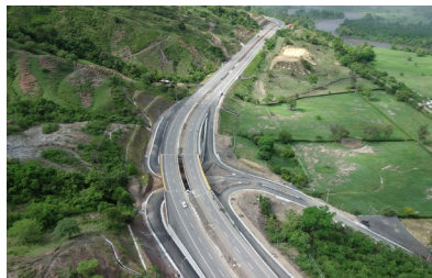
► RUTA DEL SOL SECTOR I (SECTIONS II AND III) Guaduas, Cundinamarca
