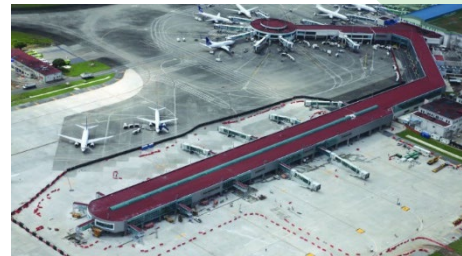
► TOCUMEN INTERNATIONAL AIRPORT Panama City, Panama
