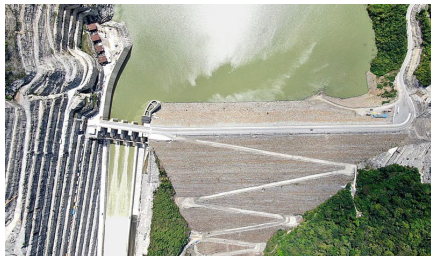
► ITUANGO HYDROELECTRIC POWER PLANT Ituango, Antioquia
