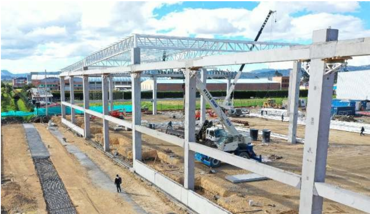
Prefabricated beam connection system. Lógica Siberia Project, Cundinamarca.
