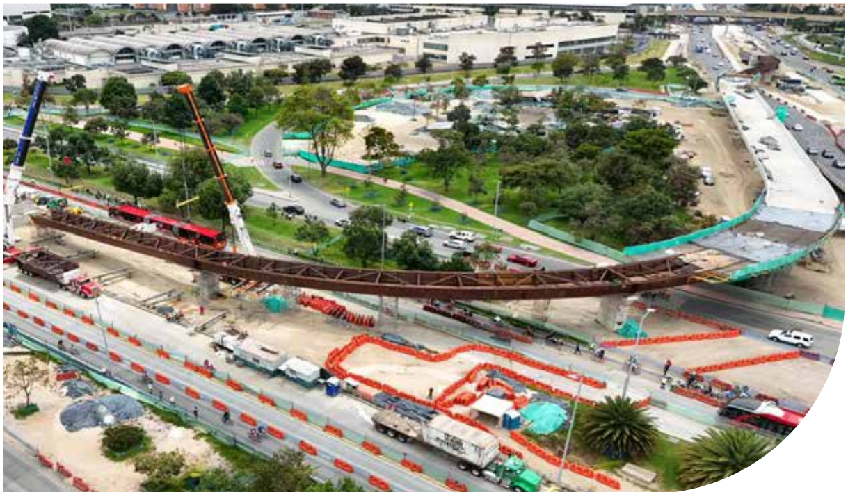
▲ Progress of the Group 5 Project, Avenida 68, Bogotá.
