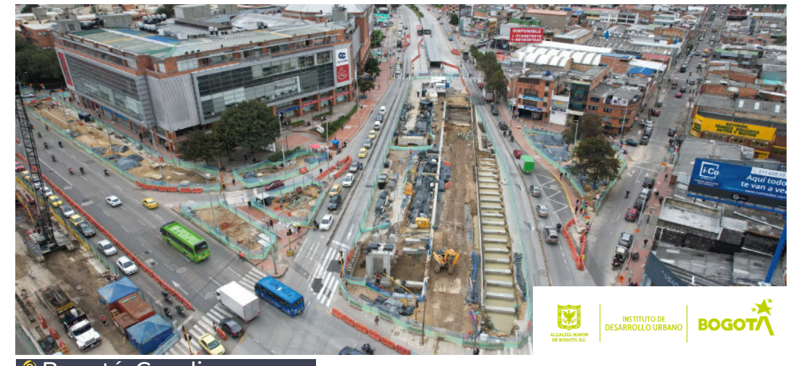
Bogotá, Cundinamarca TRANSMILENIO AVENUE 68 – GROUP 8
