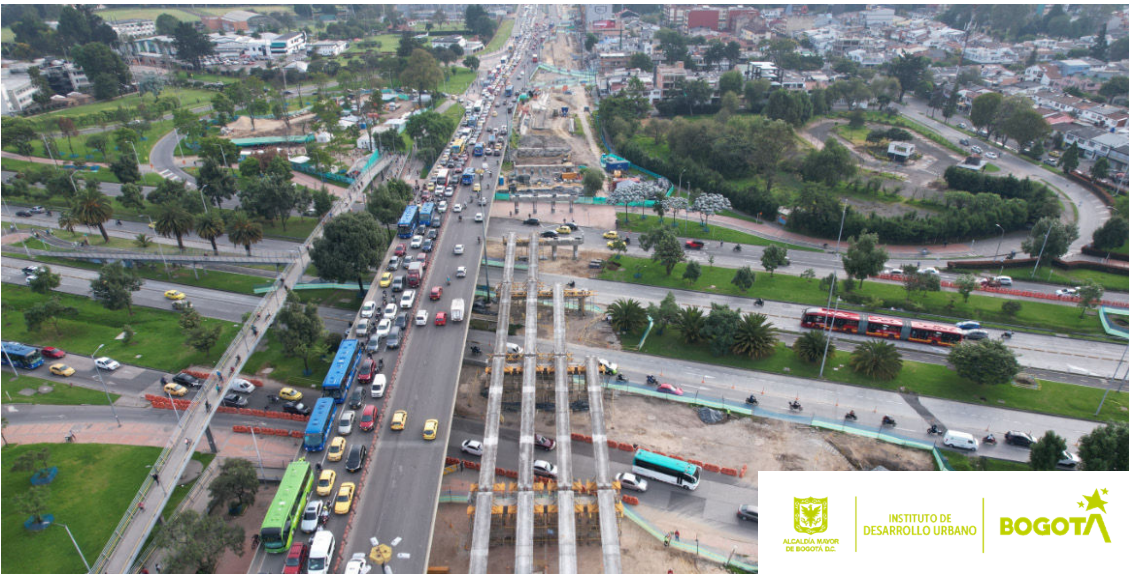
Bogotá, Cundinamarca TRANSMILENIO AVENUE 68 – GROUP 5
