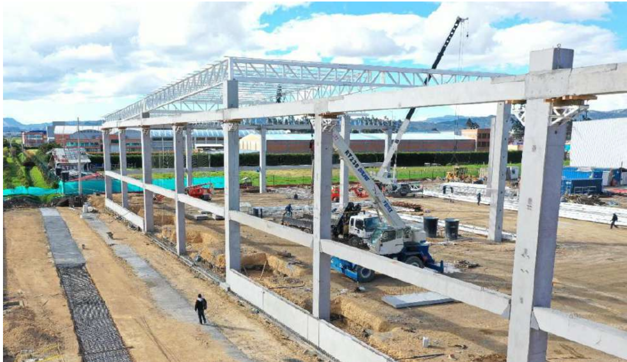
Precast beam connection system; Lógica Siberia Project, Cundinamarca
